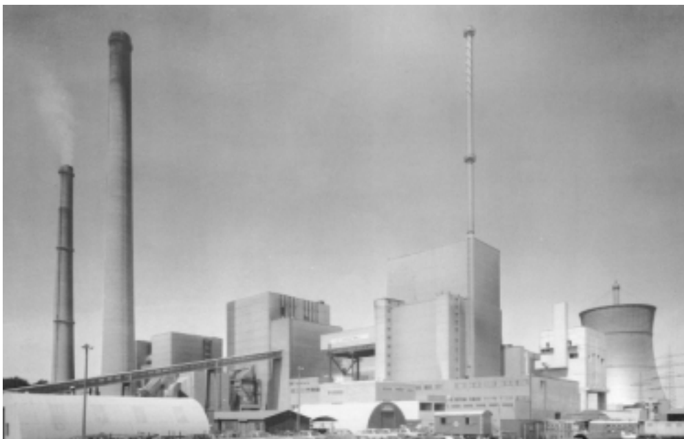
The 300-MWe THTR reactor in Germany operated between 1983 and 1989 with 674,000 pebbles, over half of them containing thorium/highly enriched uranium fuel.
